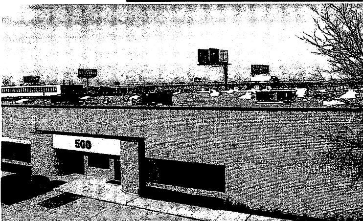
Industrial building: Modified bitumen
